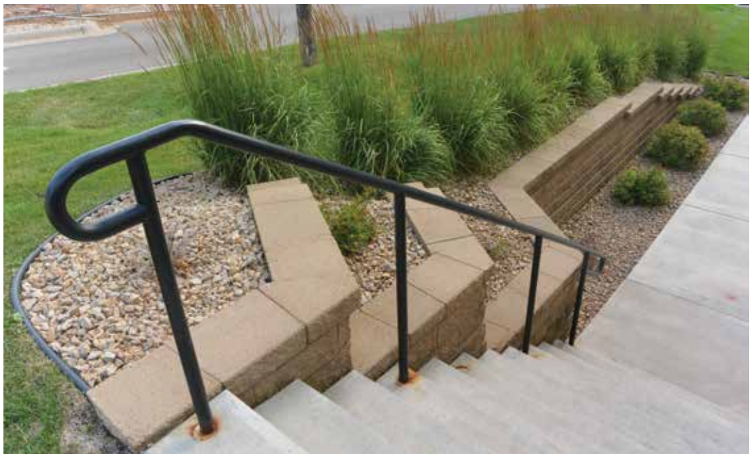
Left For the 500-foot-long wall, Landscape Reflections Inc. of Oakdale, Minn., installed 3,800 square feet of VERSA-LOK Standard units and 2,200 square yards of the manufacturer's geogrid soil reinforcement product.
