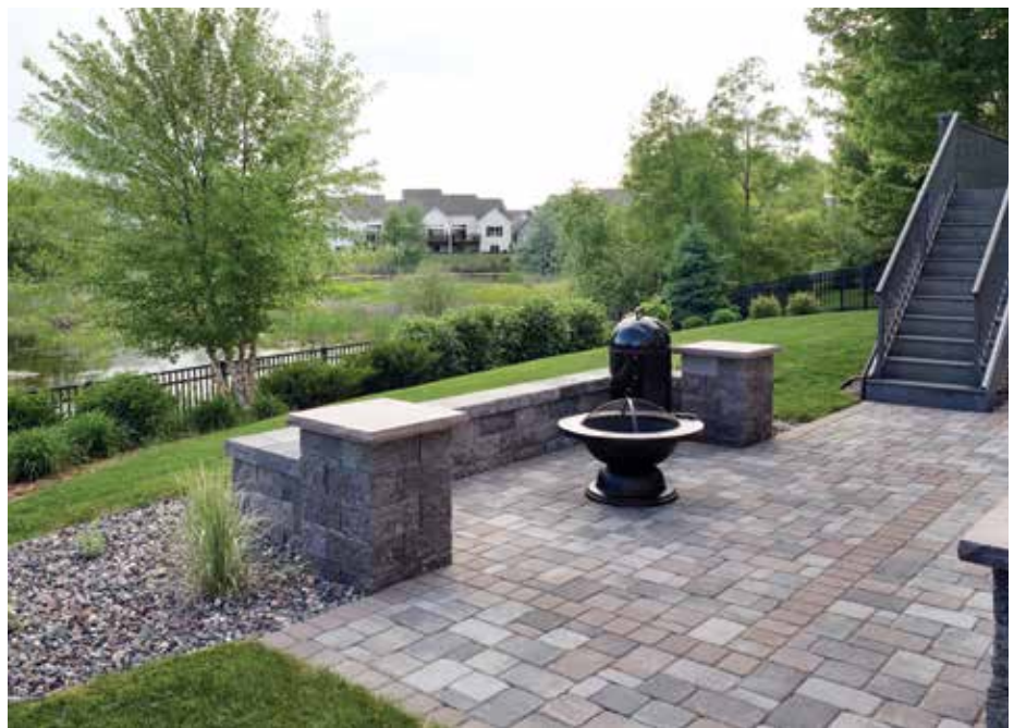
Below River rock mulch and small plants encompass the patio and incorporate elements of the existing landscaping, into the installation. A very small mulch divider keeps the river rock from being scattered about the yard. The freestanding wall, built with Standard units, adds seating for the fire pit. The columns are capped with Willow Creek Capstone in Desert brown.
