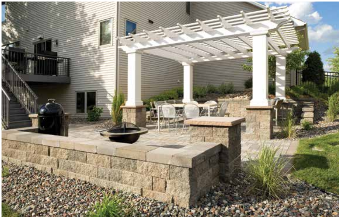
Below River rock mulch and small plants encompass the patio and incorporate elements of the existing landscaping, into the installation. A very small mulch divider keeps the river rock from being scattered about the yard. The freestanding wall, built with Standard units, adds seating for the fire pit. The columns are capped with Willow Creek Capstone in Desert brown.
